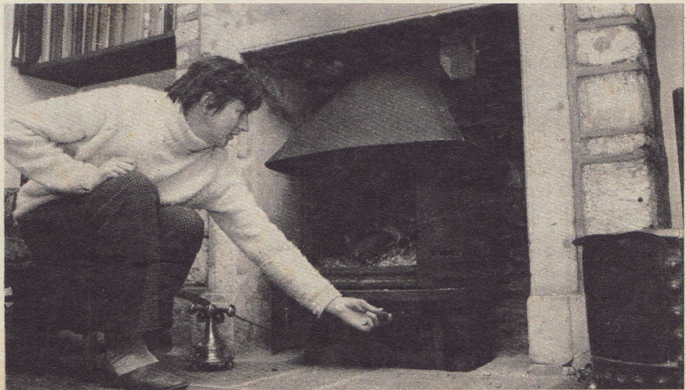
Mary Knight warms up beside the wood burning stove which has taken the shivers out of her Marshfield, Chippenham, Wilts., farmhouse. Built of cast iron it is fitted with doors which enclose the fire completely at night and keep it safely smouldering until morning. With the doors and draught vents open the fire quickly blazes into life.
